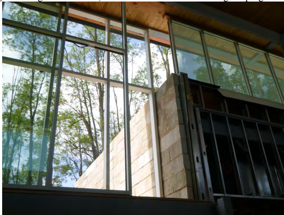
Project Site on August 28, 2018 Curtain wall above zig zag seating area.
