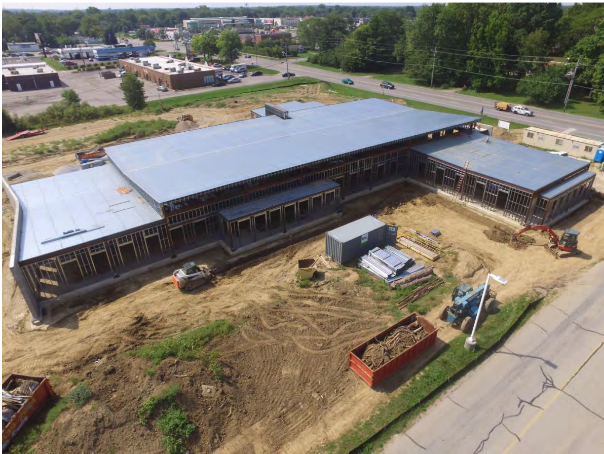
Project Site on September 4, 2018 View looking southwest.
