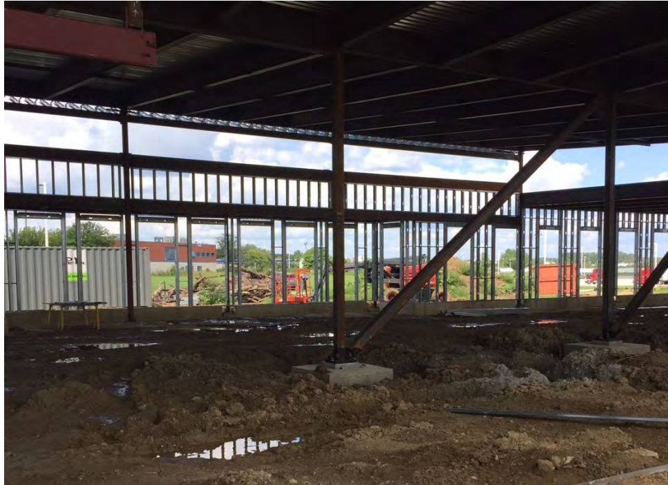
Project Site on August 22, 2018 View looking northeast showing the windows in the Teen's Area.
