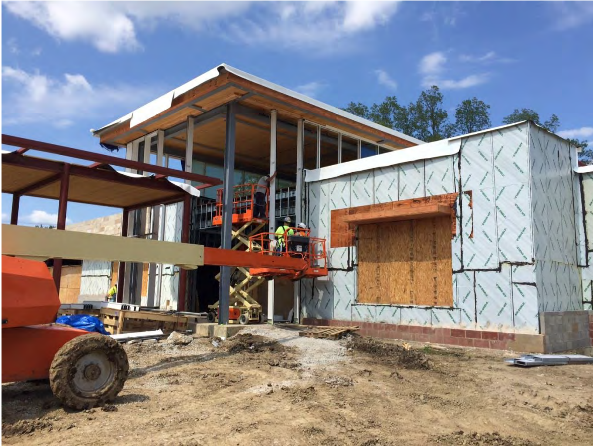
Project Site on August 28, 2018 View of the entry canopy and the concourse roof.
