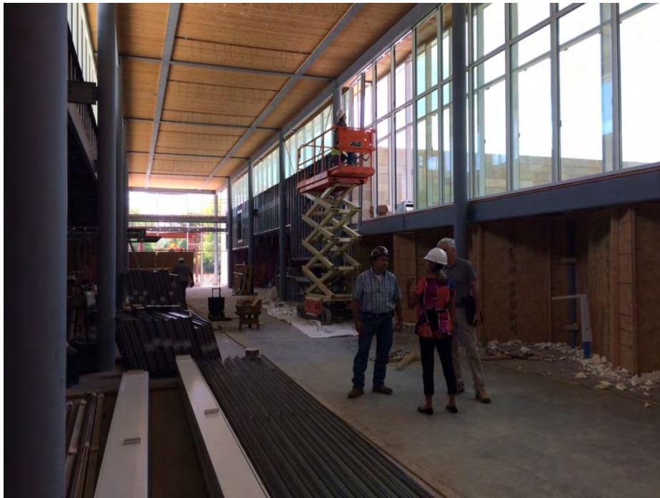
Project Site on August 28, 2018
