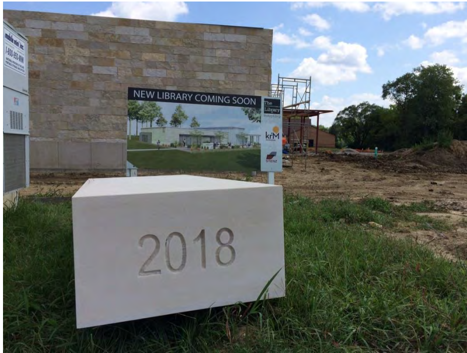
Project Site on August 28, 2018
